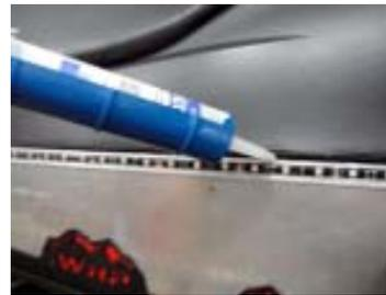
Final step on any exposed surface LED, use a 100% clear silicone bead on the entire length of the strips and ends.
